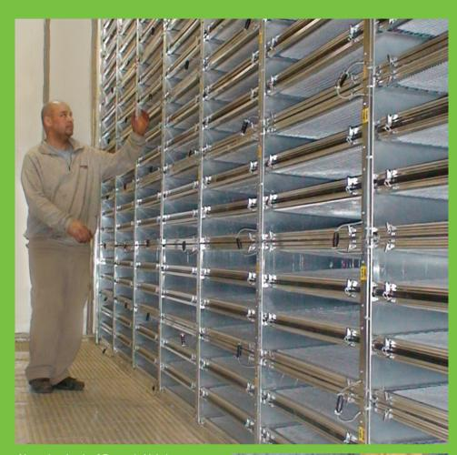
Above is a bank of Dynamic V8's in a 125,000 cfm custom air handler in a high-risk office application. These units are permanently mounted with front access.
